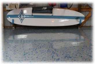
**GARAGE FLOOR PC-149 EPOXY PRIMER CM-15 EPOXY MASTIC** CT-332 CLEAR
