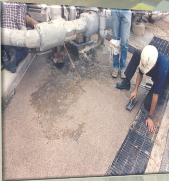
PC-1000 Epoxy Mortar used for resurfacing concrete in containment area.
