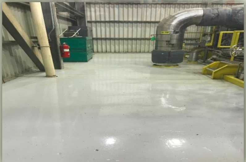
PC-1850 100% Solids Epoxy used in a turbine room.
